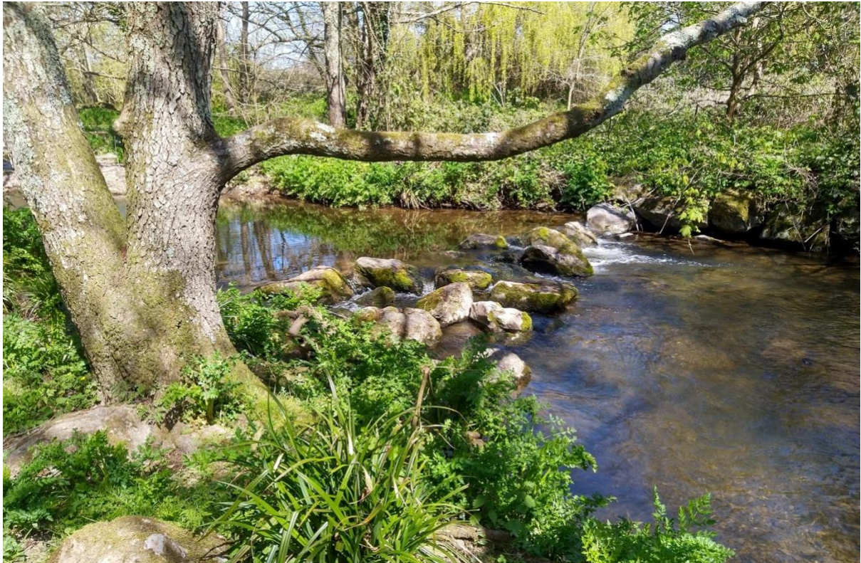
Figure 3 The first boulder weir immediately upstream of another at Figure 4. This should be altered with an aim to provide general roughness, over the appearance of a weir. SY 13304 88965
