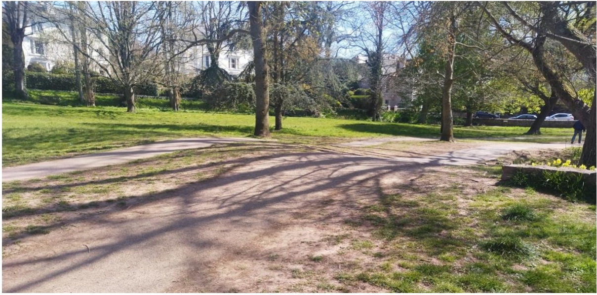
Figure 27 The bund next to School Weir, designed to hold back flood water into the upper Byes. SY 12790 87895
