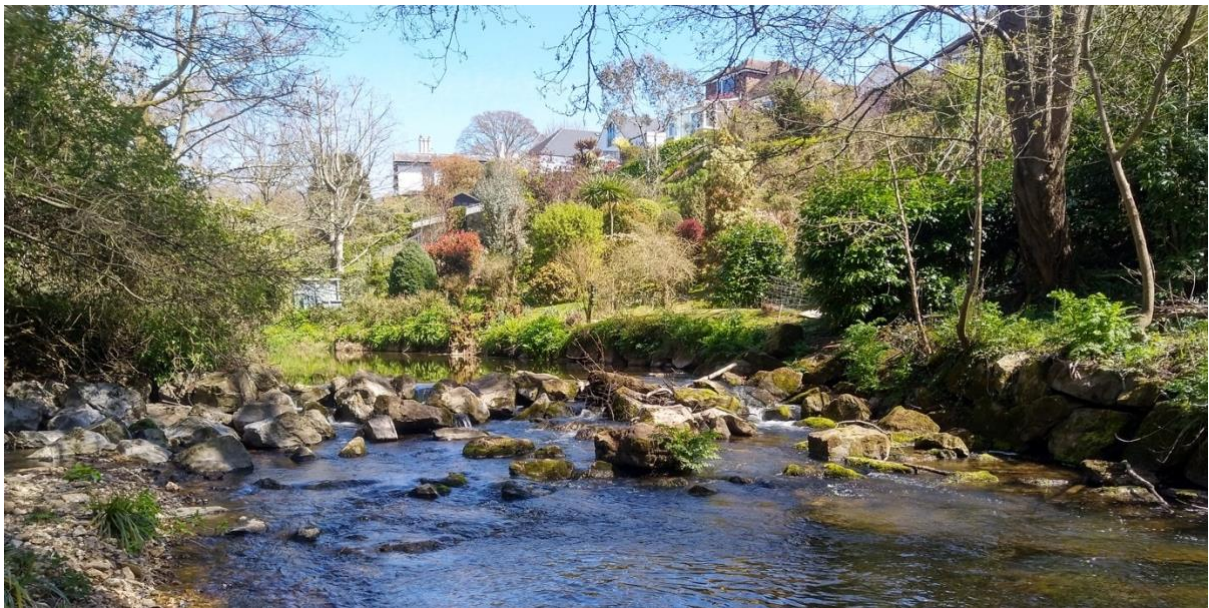
Figure 10 Easing of this boulder weir will increase the pace of flow in the impoundment by the gardens (as seen in Figure 9). Work will be needed to prevent erosion of their banks, but the river course could be encouraged toward the RB. SY 13171 88701
