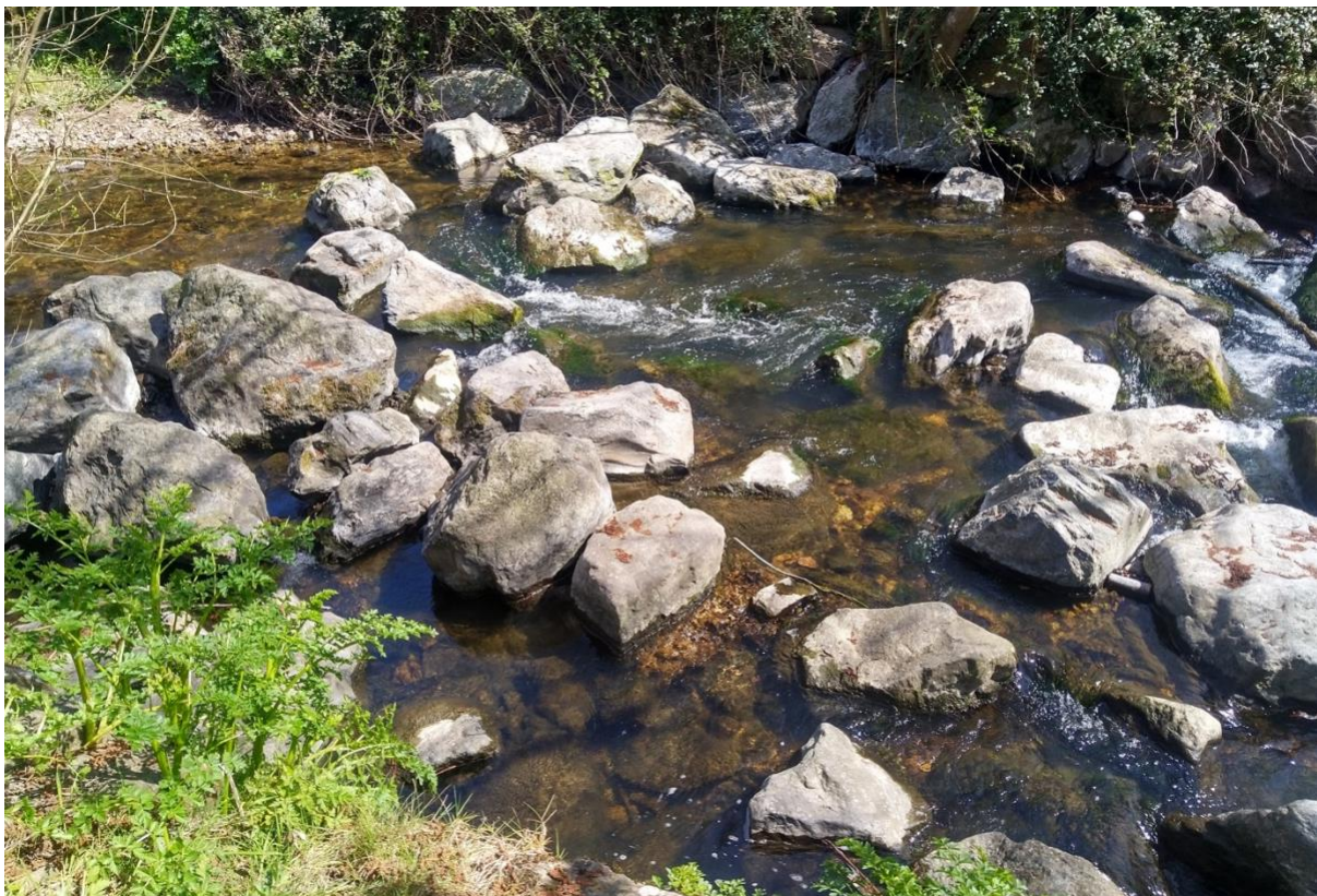
Figure 22 Directly downstream of Figure 20, another reasonable rubble weir. Again, this could be made redundant (at least partially) through meandering. SY 12852 88305
