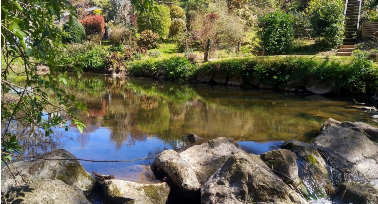
Figure 9 Another boulder weir. Note the impoundment of the river above and the stone revetment of the garden banks. This calm water may be seen as desirable for the bankside gardens but is detrimental for the habitat. SY 13171 88701
