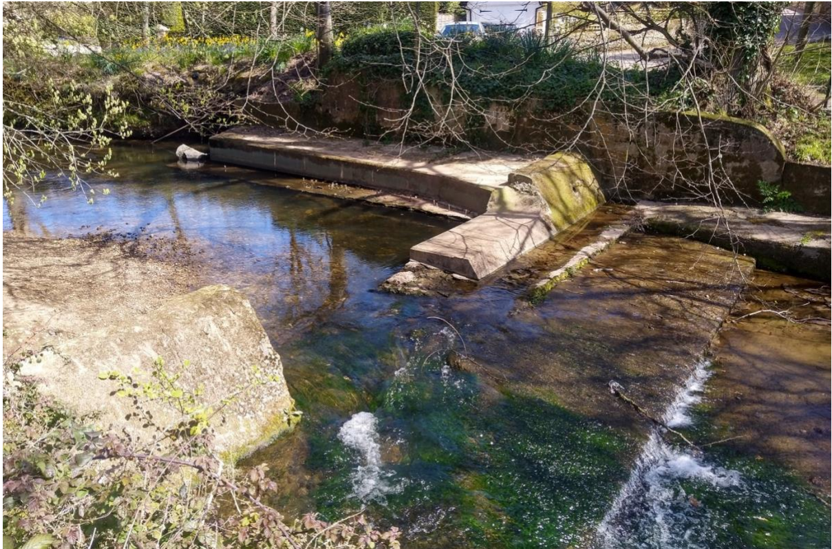
Figure 17 Another old weir that has had a section removed. Despite this improvement for fish passage, the three shallow steps downstream are a significant impediment to fish passage. Total removal would be the best course of action. SY 12969 88498
