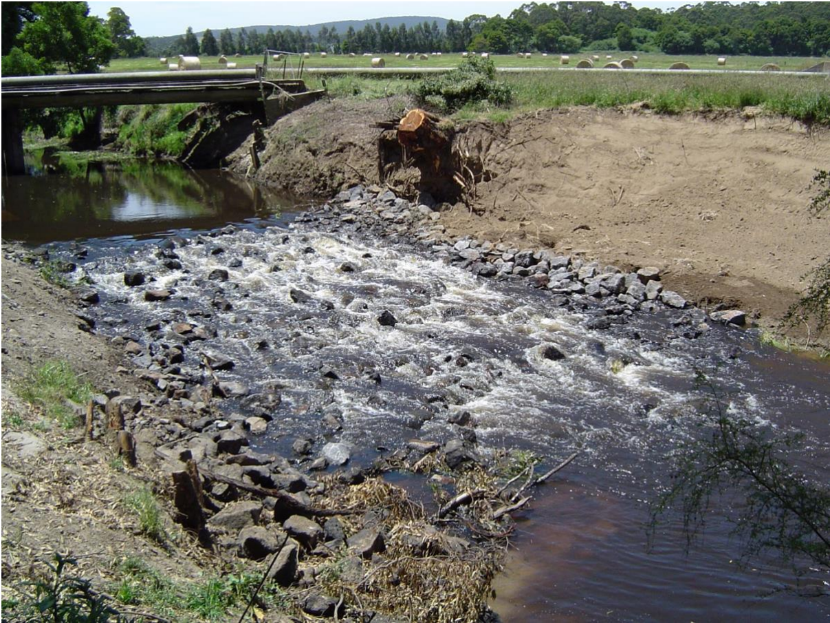
Figure 30 A rock ramp installed on an impassable weir.
