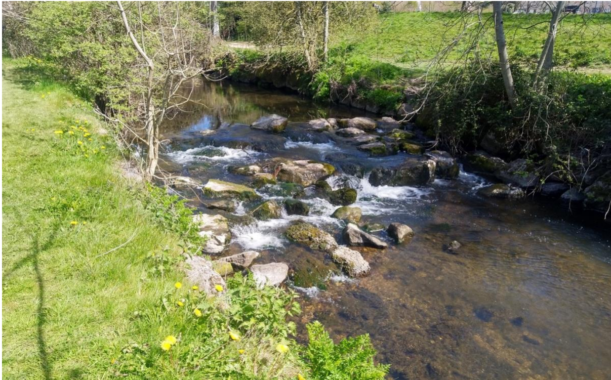
Figure 21 A better looking rubble weir, though still an unnecessary impediment to natural river function and fish migration. With room on both banks, the gradient could be reduced through meandering rather than an unnatural step. This would restore a lateral scour pool and riffle sequence, good for all salmonid life stages. SY 12863 88312
