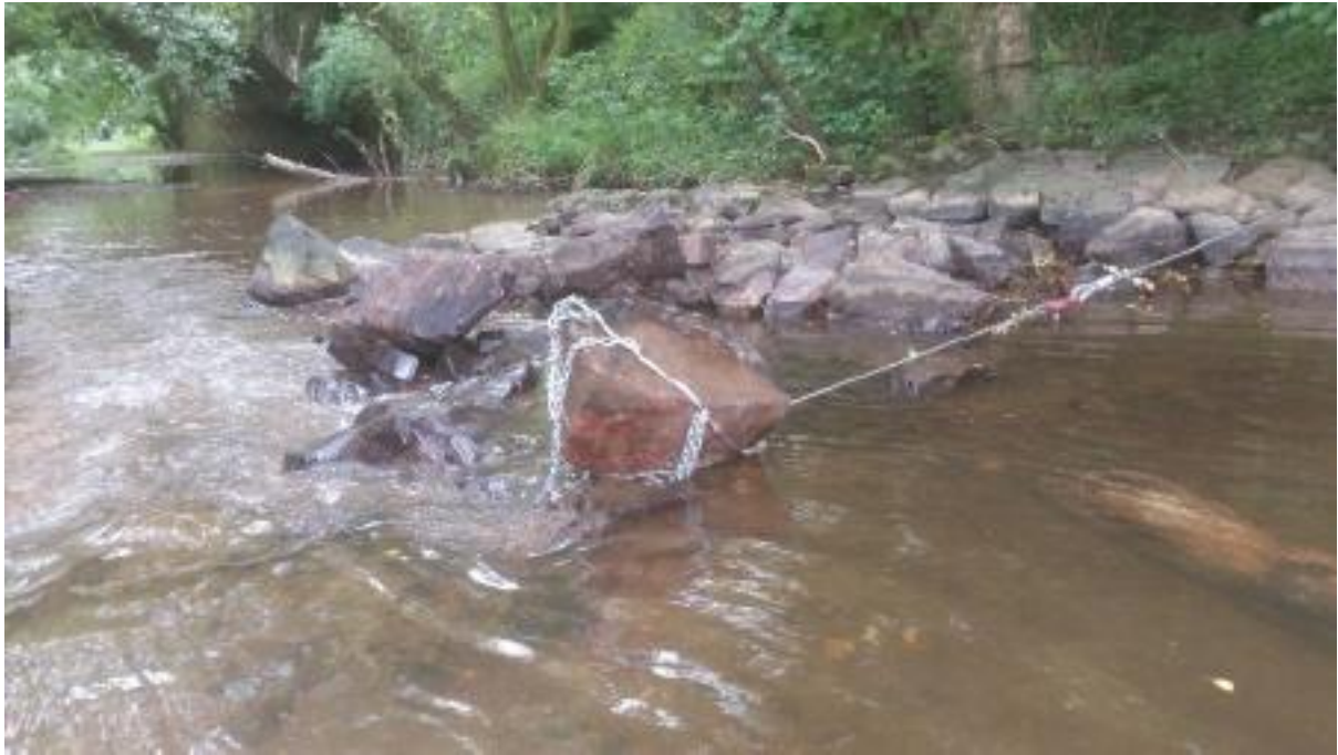
Figure 32 The winch sling in action on the River Yeo, near Crediton, Devon.
