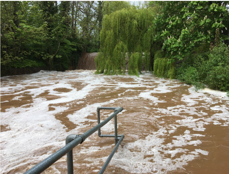
School Weir 13th May 2021 after heavy rain
