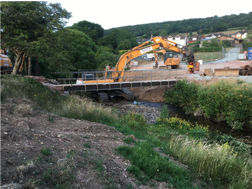
Photo 6 Fortescue Bridge works
